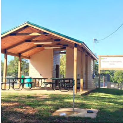
2B Restrooms / Shower / Picnic Pavilion
