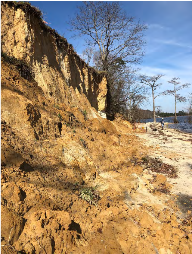
TGOW SITE EXISTING CONDITIONS - VIEW FROM BEACH TOE OF BLUFF
