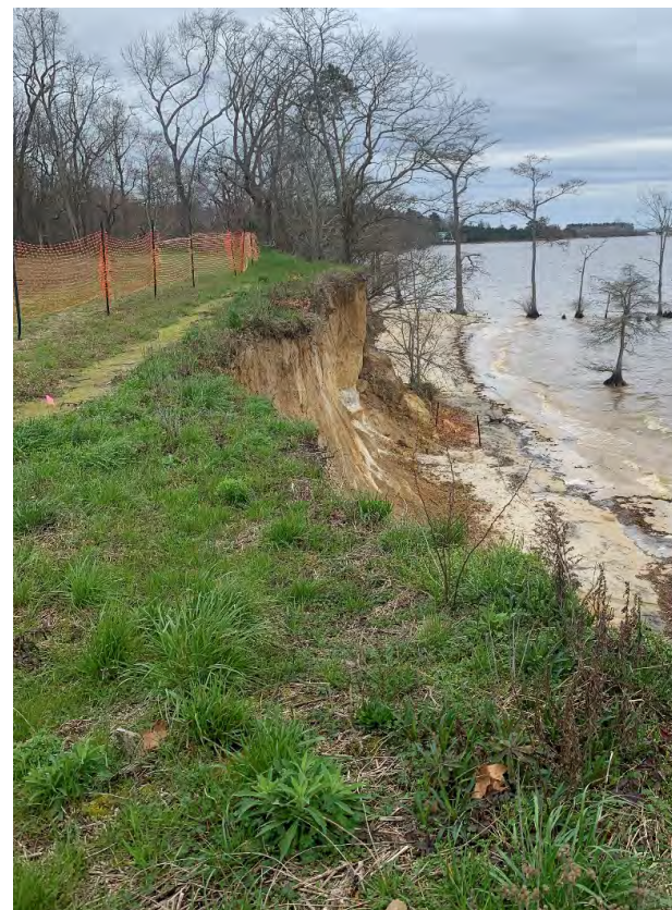
TGOW SITE EXISTING CONDITIONS - VIEW FROM TOP OF BLUFF
