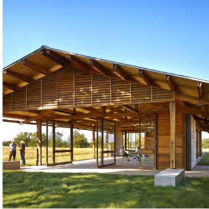
4C Restroom / Shower / Picnic Pavilion
